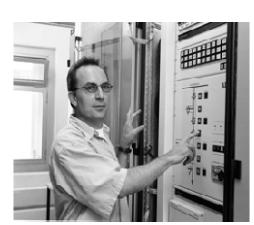
Sometimes, the group level has its own man-machine interface for local operation control (here: cement packaging)
