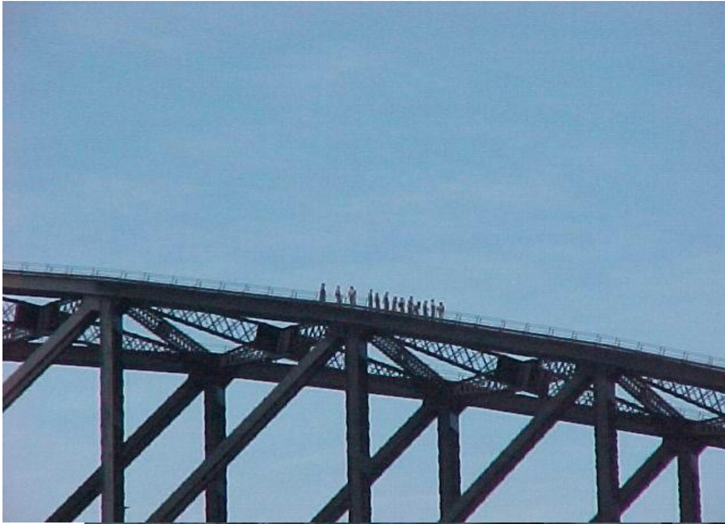
Sydney Harbour Bridge, Sydney, Australia
